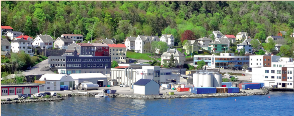
Marine Ingredients' processing plant in Brattvaag currently employs nearly 50 people.
