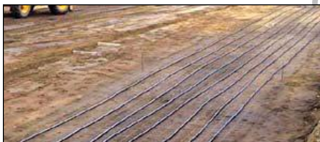
Figure 4.38: Example of PE pipes ready to be cast in concrete
