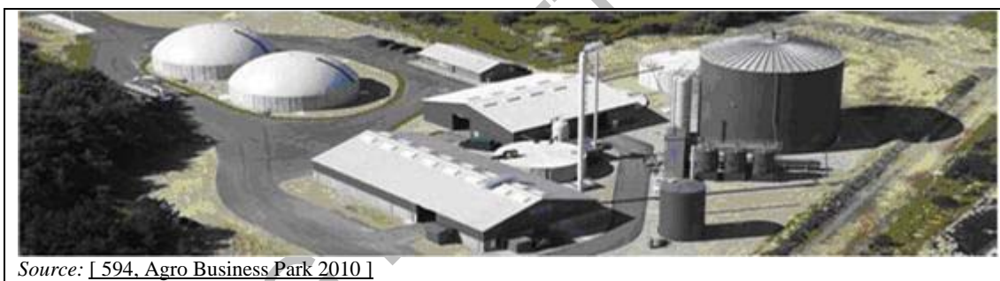
Figure 4.82: Example of biogas installation, from anaerobic treatment of manure, located in Denmark
