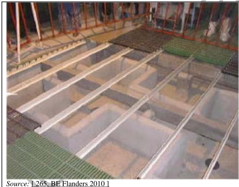
Figure 4.53: Shallow slurry pits separating manure and water channels during construction
