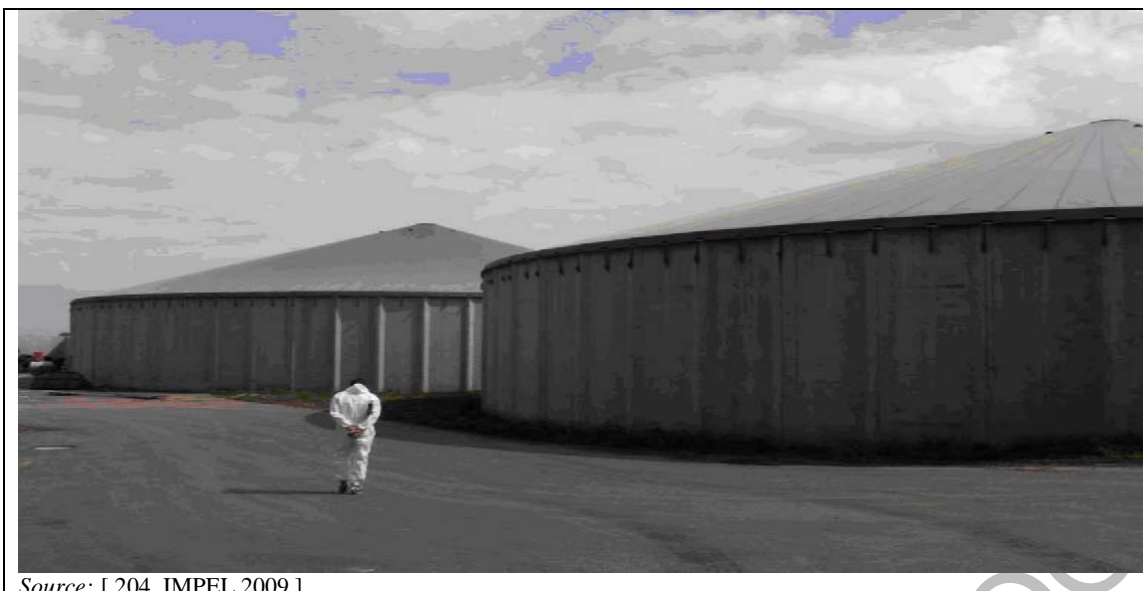
Figure 4.71: Rigid cover for slurry storage, with conical shape
