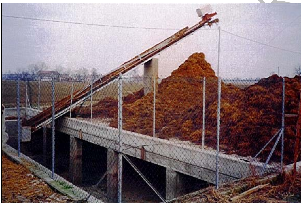
Figure 2.34: Storage of littered manure with separate containment of the liquid fraction (Italy)
