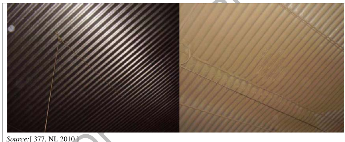
Figure 2.10: Effect of dust attraction caused by ionisation on the roof of a poultry shed
